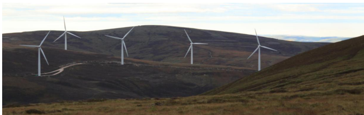
Figure 4 - Backclothing of wind turbines due to elevated view in addition to visibility against hill behind
