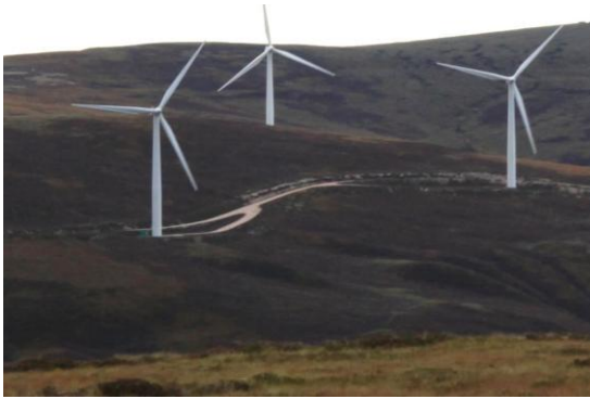
Figure 6a – wind turbine tracks contrast to dark vegetation background (Photograph taken 8 years after commissioning)
