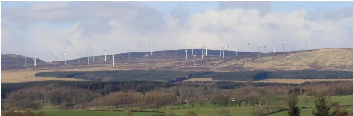
Figure 3 - Backclothing of turbines due to location of windfarm upon hill side slopes
