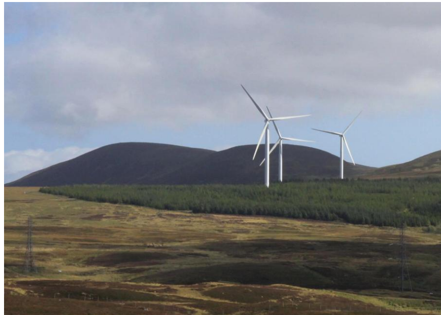
Figure 20 - Differing colour contrast of wind turbines between a sky background and a hill background (this can be compared to the colour contrast of high voltage powerlines in front)
